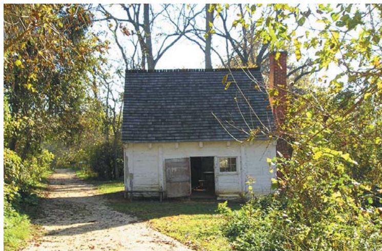
Figure 33: Current view of Sotterley's slave cabin
