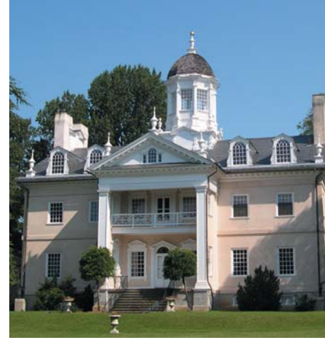
Figure 37: Current lawn entrance view of Hampton
